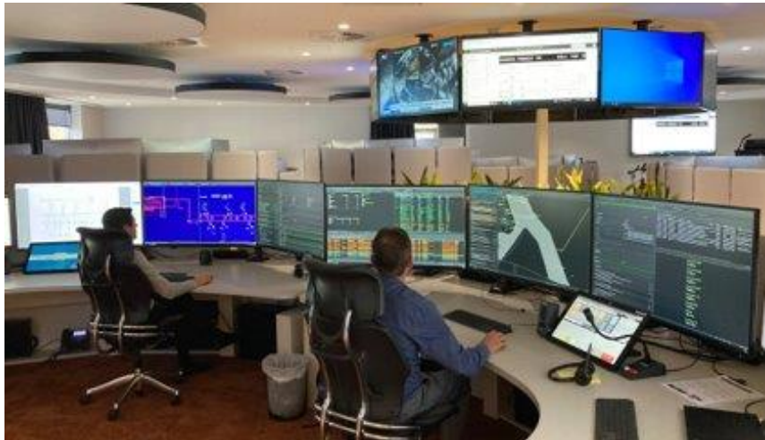
New Control Room fit-out
